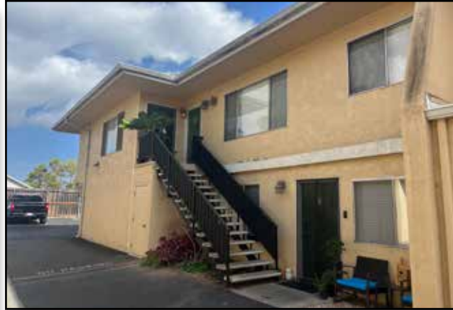
North Side of Building Driveway to Parking in Rear
