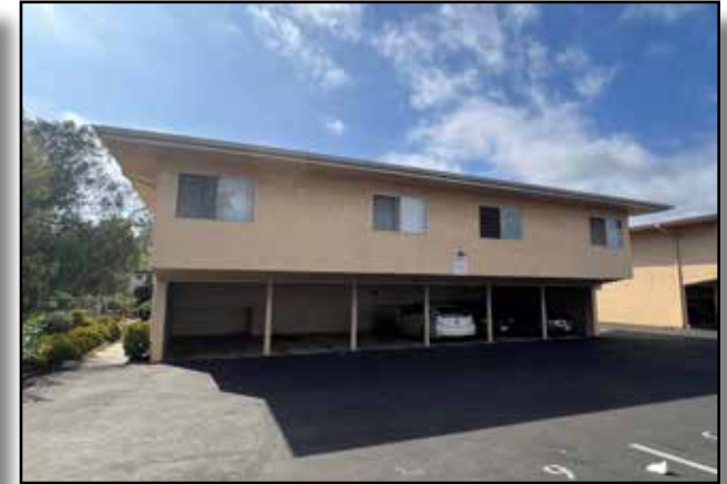
6 Carport Spaces, Plus Storage 8 Uncovered Spaces at Back
